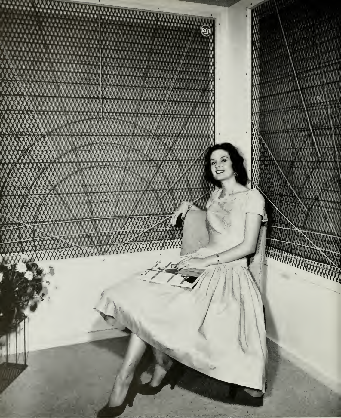
Inside the world's first electronically air conditioned room, at RCA's David Sarnoff Research Center. Cooling or heating are provided noiselessly by wall panels behind decorative grills shown here.
